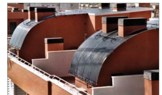
Unglazed collector using liquid transfer medium
